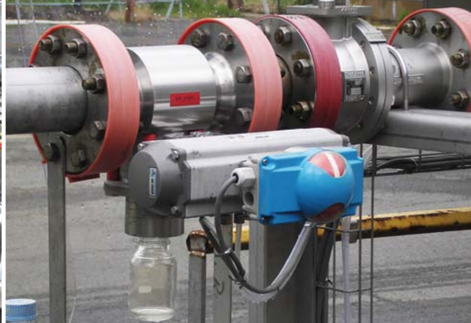
Sampling of acid for quality control
