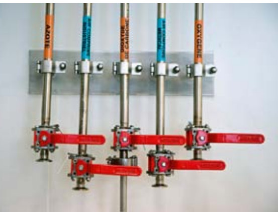
Valves with welded and clamp connections in a research laboratory
