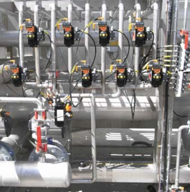
Valves with actuators on agrochemical process
